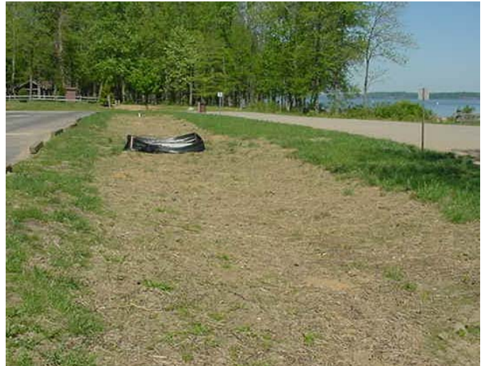
Photo of bioretention area following construction, April 2004.
