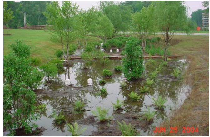
Photograph of the bioretention demonstration project taken during a rainfall event in June 2004.
