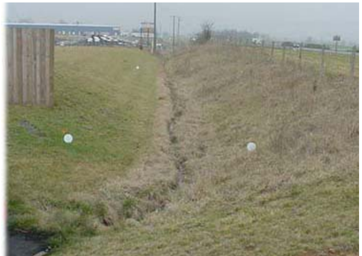
Above: The ditch where the rain garden was later constructed.
