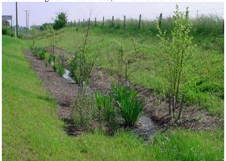
Below: Rain garden in June 2003, 14 months after construction.
