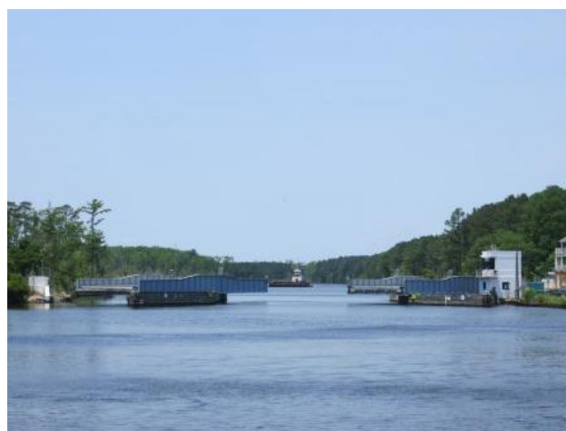
Figure 3-22. Existing North Landing Bridge, facing north. (Source: USACE)
