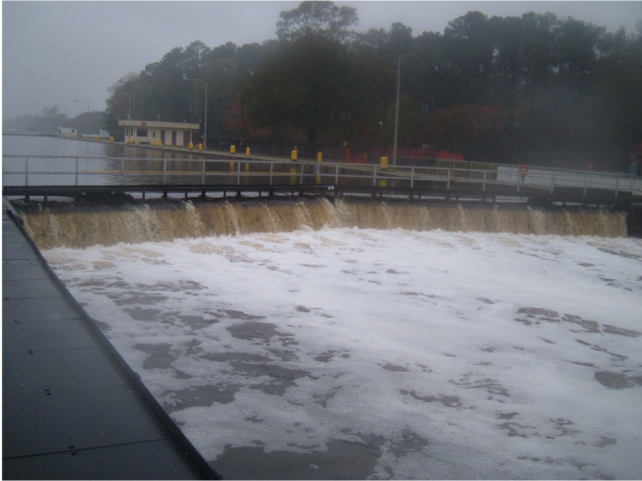
Figure 3-9. Great Bridge Lock – 2009 Nor'Ida Event.
