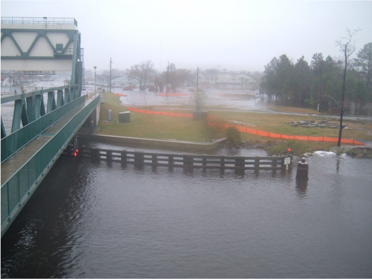
Figure 3-10. Great Bridge Bridge – 2009 Nor'Ida Event.
