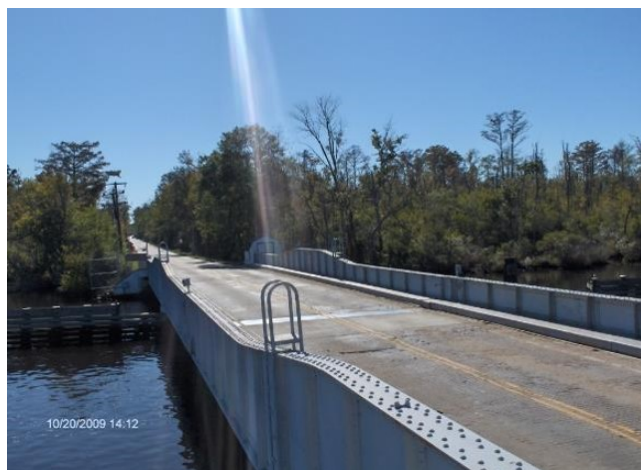
Figure 3-23. Existing North Landing Bridge, facing west. (Source: USACE)
