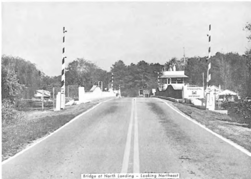
Figure 2-1. Picture of North Landing Bridge in 1976.
