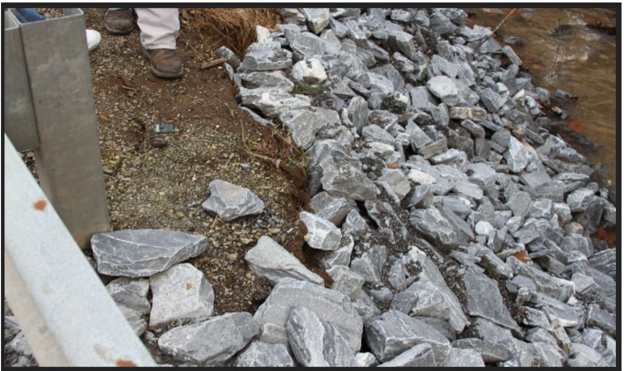
Figure 1-4. View showing riprap "slump" due to improperly designed and placed protection.
