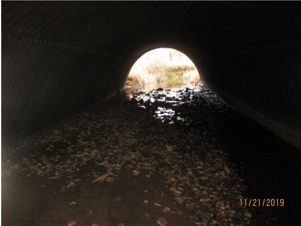
Figure 3.10 Looking downstream inside corrugated metal pipe. Gravel and soil deposits inside pipe.
