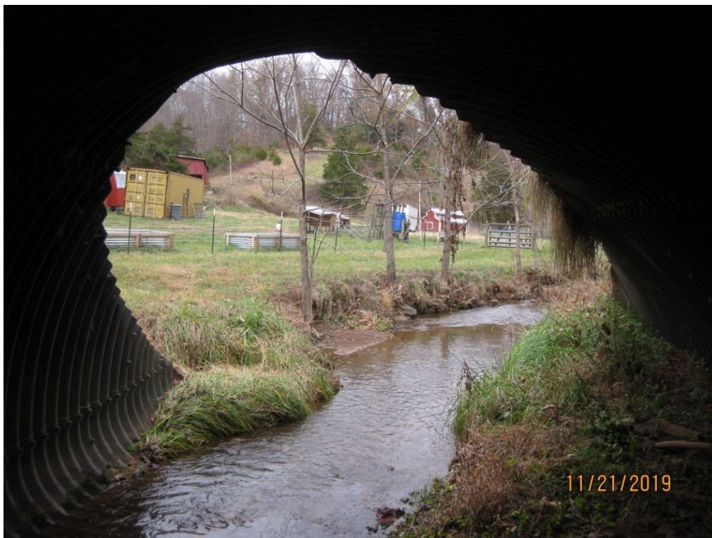
Figure 3.11 Looking downstream at corrugated metal pipe exit. Vegetation growth on sides of pipe.
