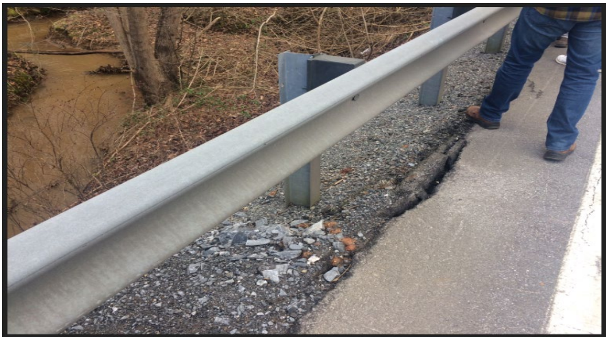
Figure 1-2. View showing roadway degradation which occurred prior to emergency slope repair.
