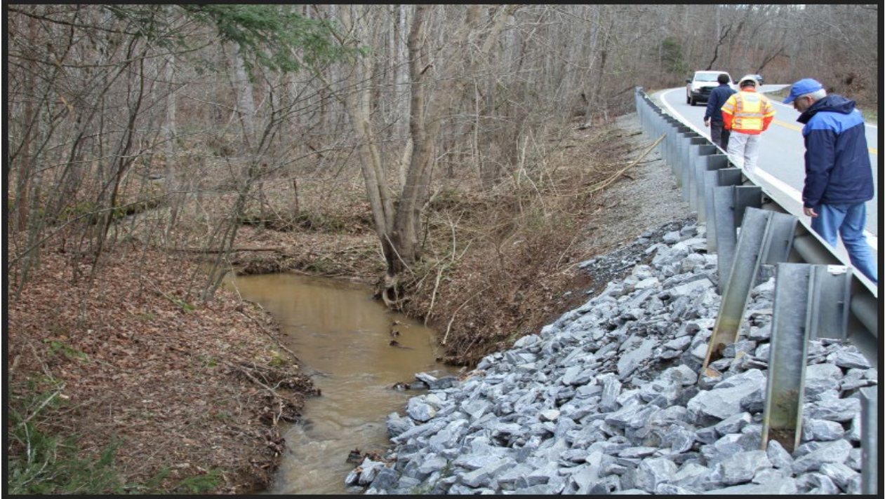
Figure 1-3. View showing roadway degradation which occurred prior to emergency slope repair.
