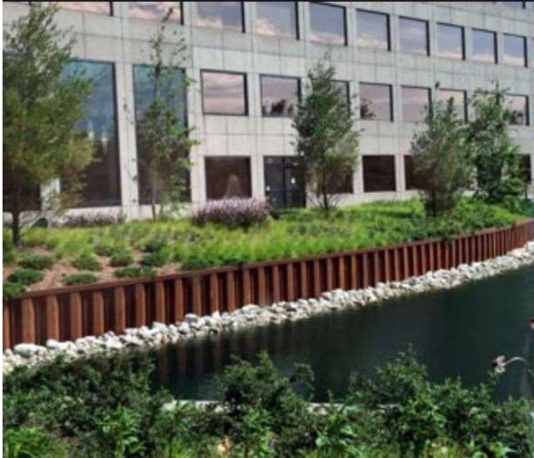
Figure 2.3 Sheet Pile Wall with Armor Stone Toe Protection
