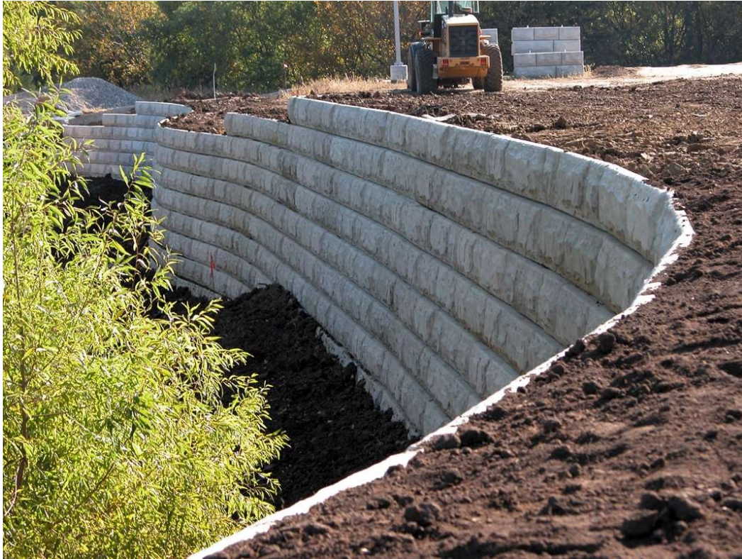
Figure 2.2 Modular Retaining Wall with Armor Stone Toe Protection
