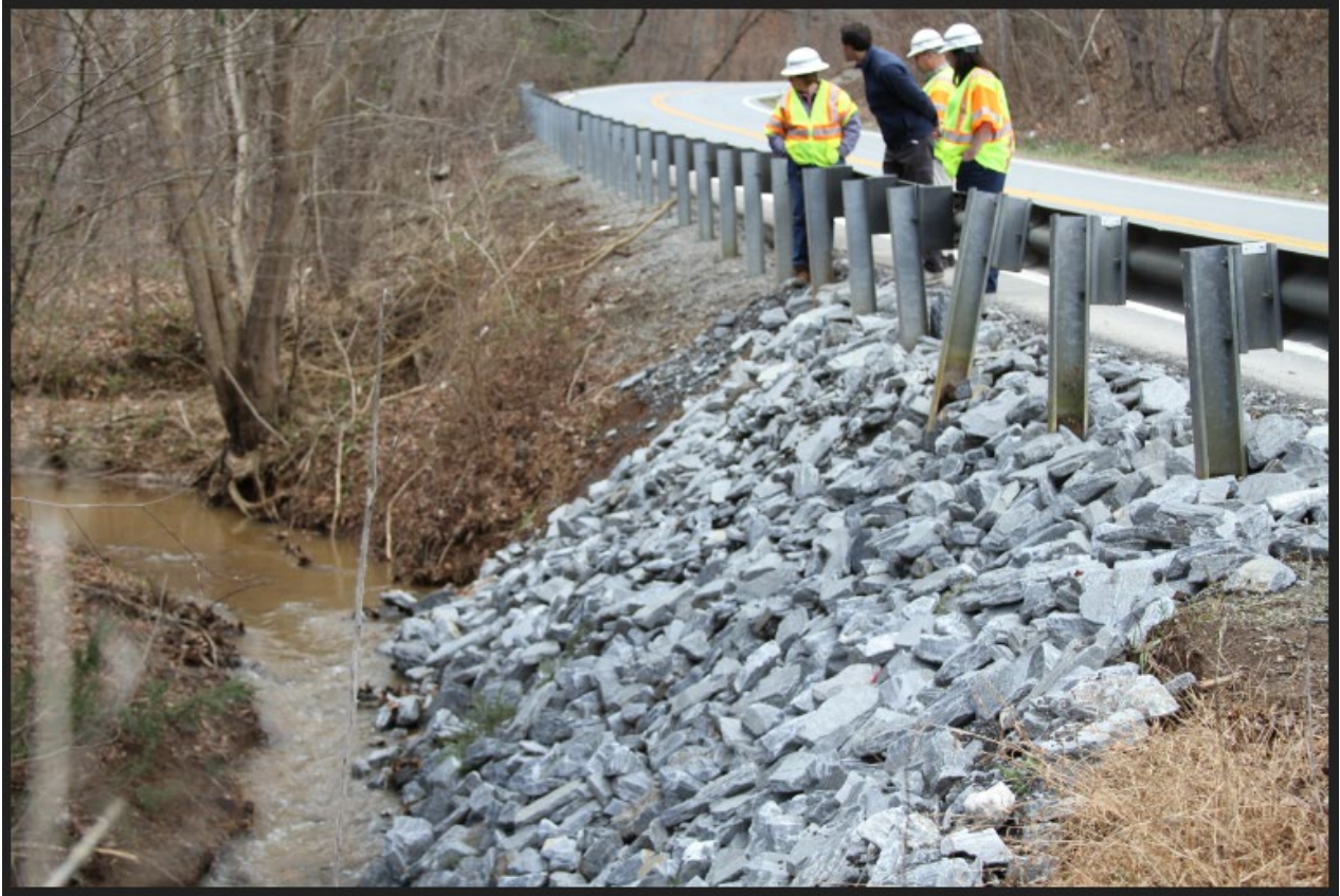
Figure 1-5. View showing riprap “slump” due to improperly designed and placed protection
