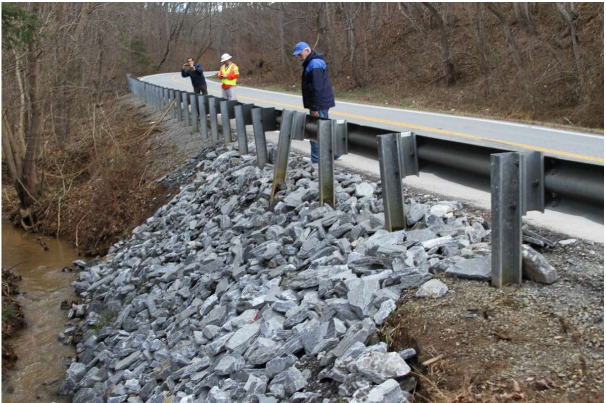
Figure 3.1 Highway embankment with Class I riprap.
