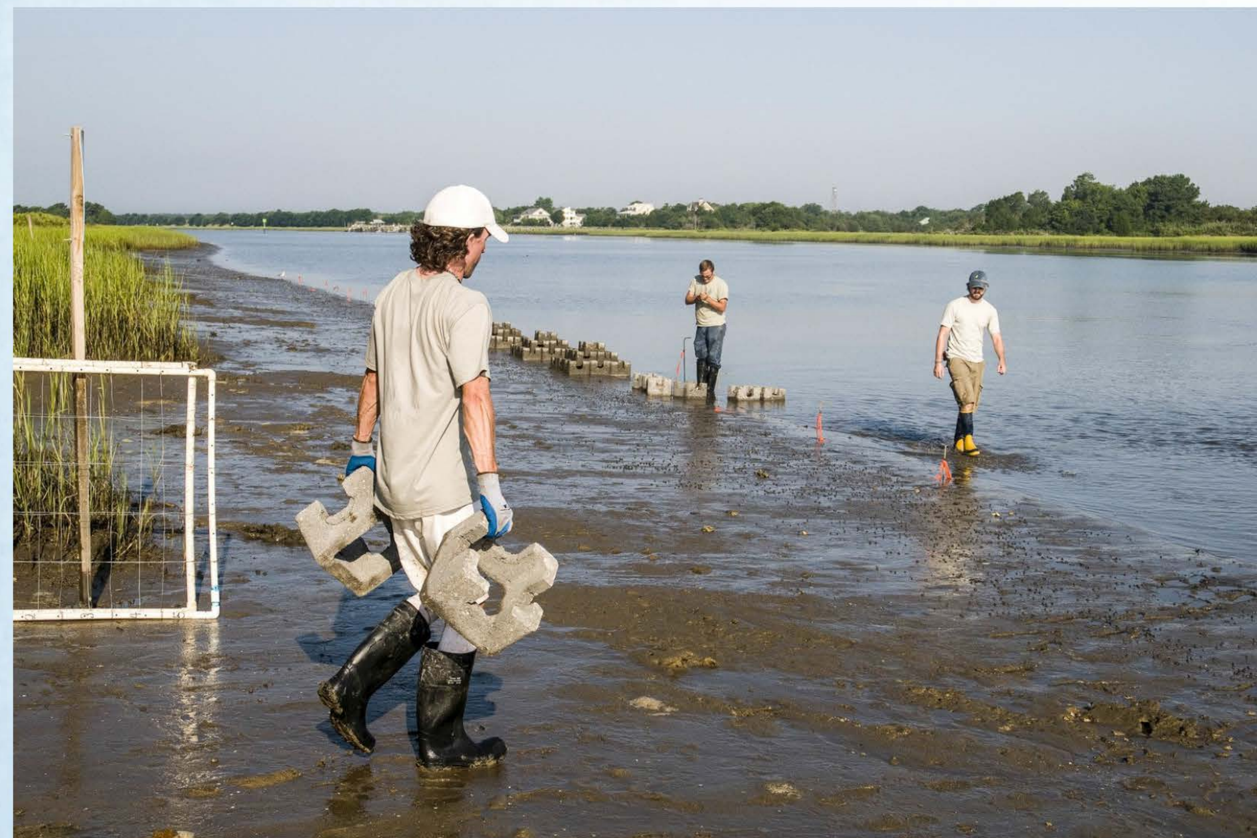
Installation of artificial reef structures
