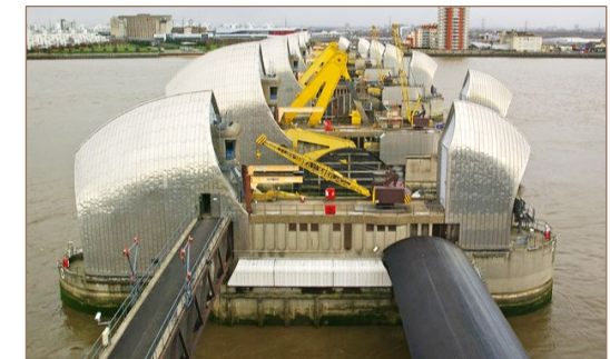
Example of existing rising sector gates at the Thames Barrier in London
