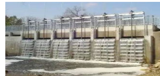
Example of Sluice gates
