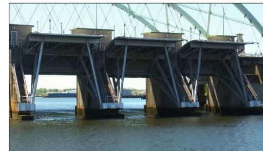
Example of existing Tainter gates at Fox Point Hurricane Barrier in Providence, Rhode Island
