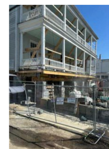
Building elevation in process
