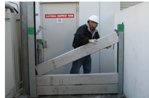
Deployable stop logs to protect vulnerable entryways
