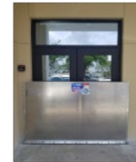
Temporary flood panels
