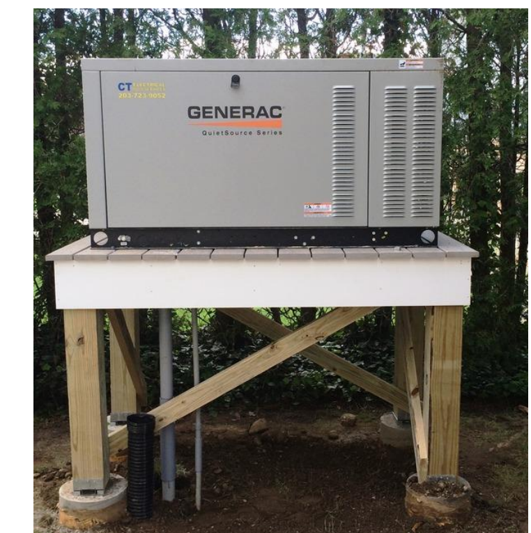
Elevated critical equipment
