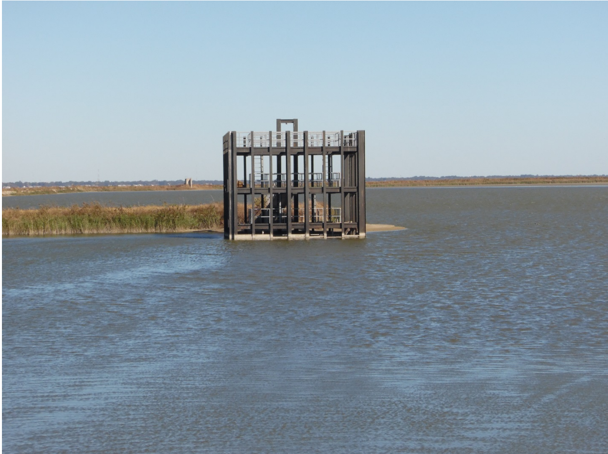
Figure 6-5. Spillway Structure - Containment Area
