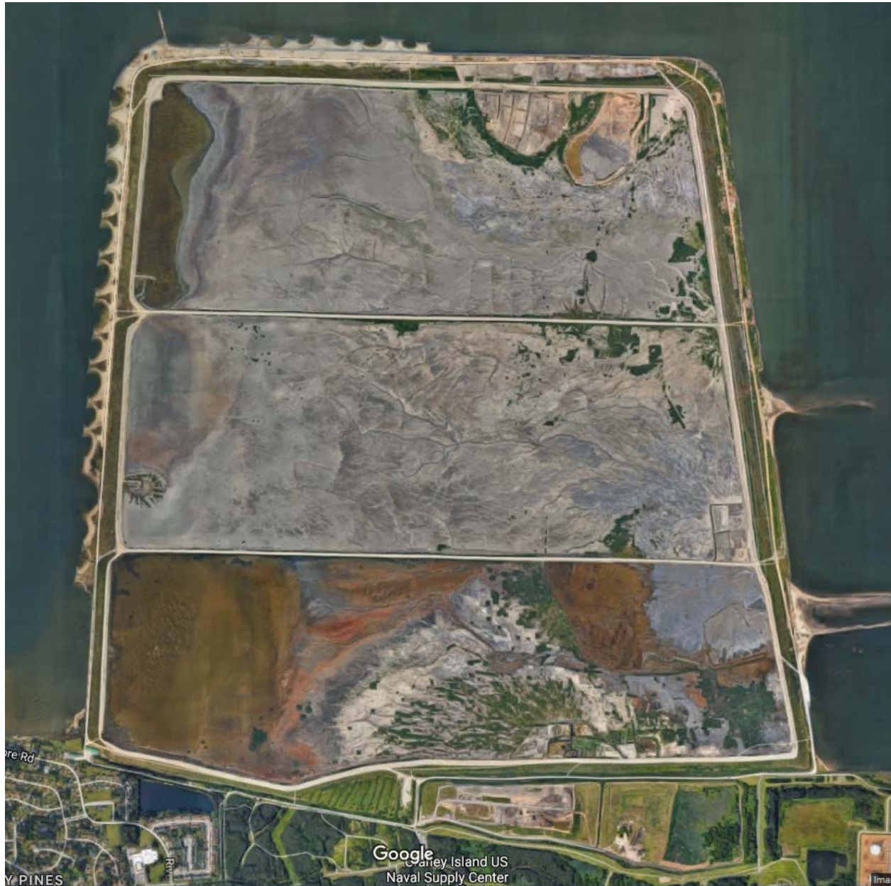
Figure 6-4. Aerial View of Craney Island Breakwater Structure
