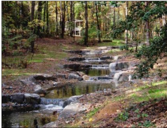
Photo 6. Step pool example (after construction).
