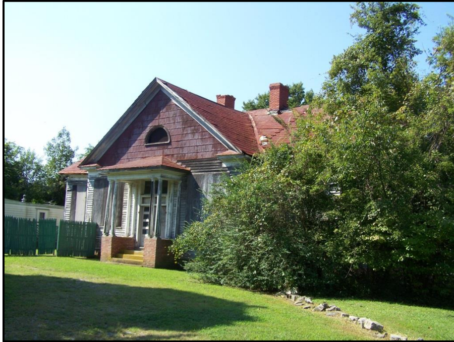
Figure 17. Bay View School (VDHR #046-5138), 6114 Old State Highway, View Looking Southwest.
