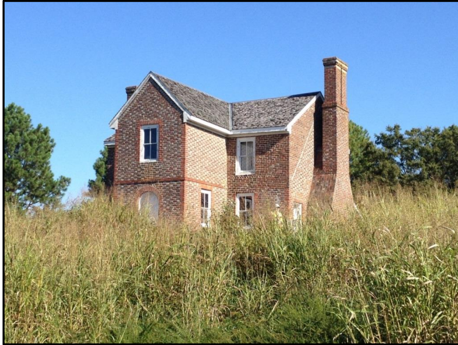
Figure 64. Matthew Jones House (Fort Eustis; VDHR #121-0006), View Looking North.
