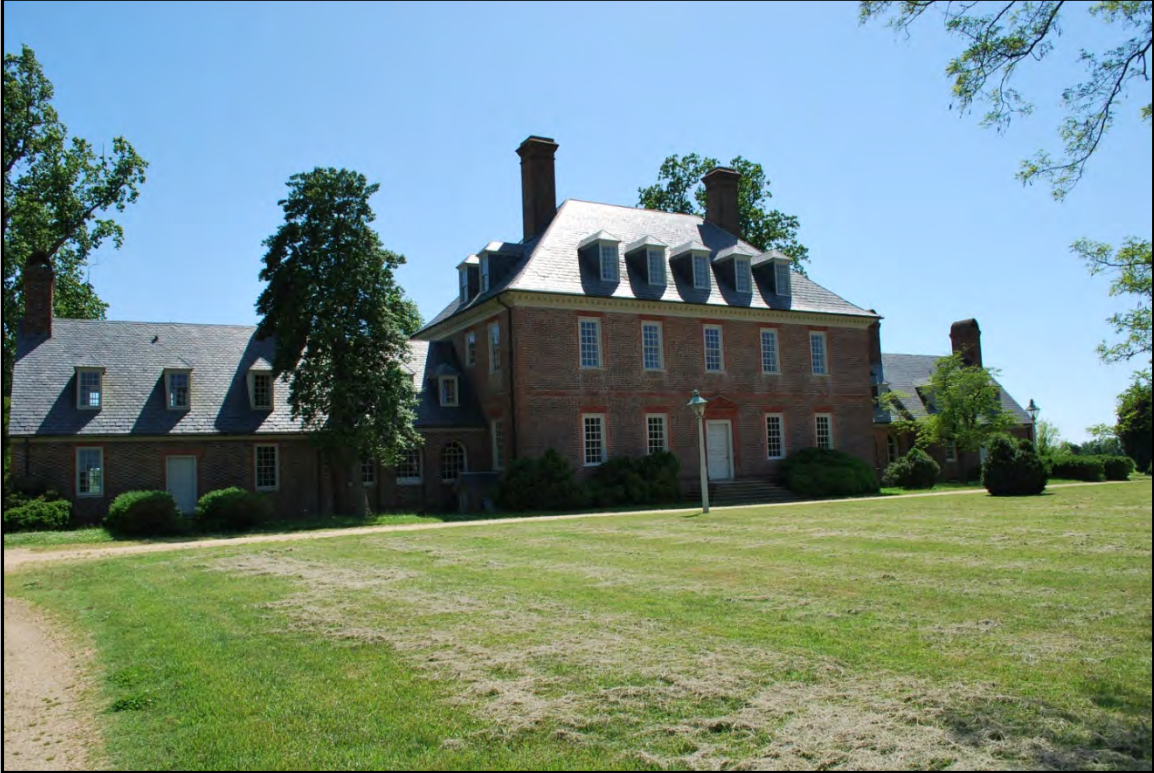
Figure 9. Carters Grove (VDHR #047-0001), Facing Southwest.
