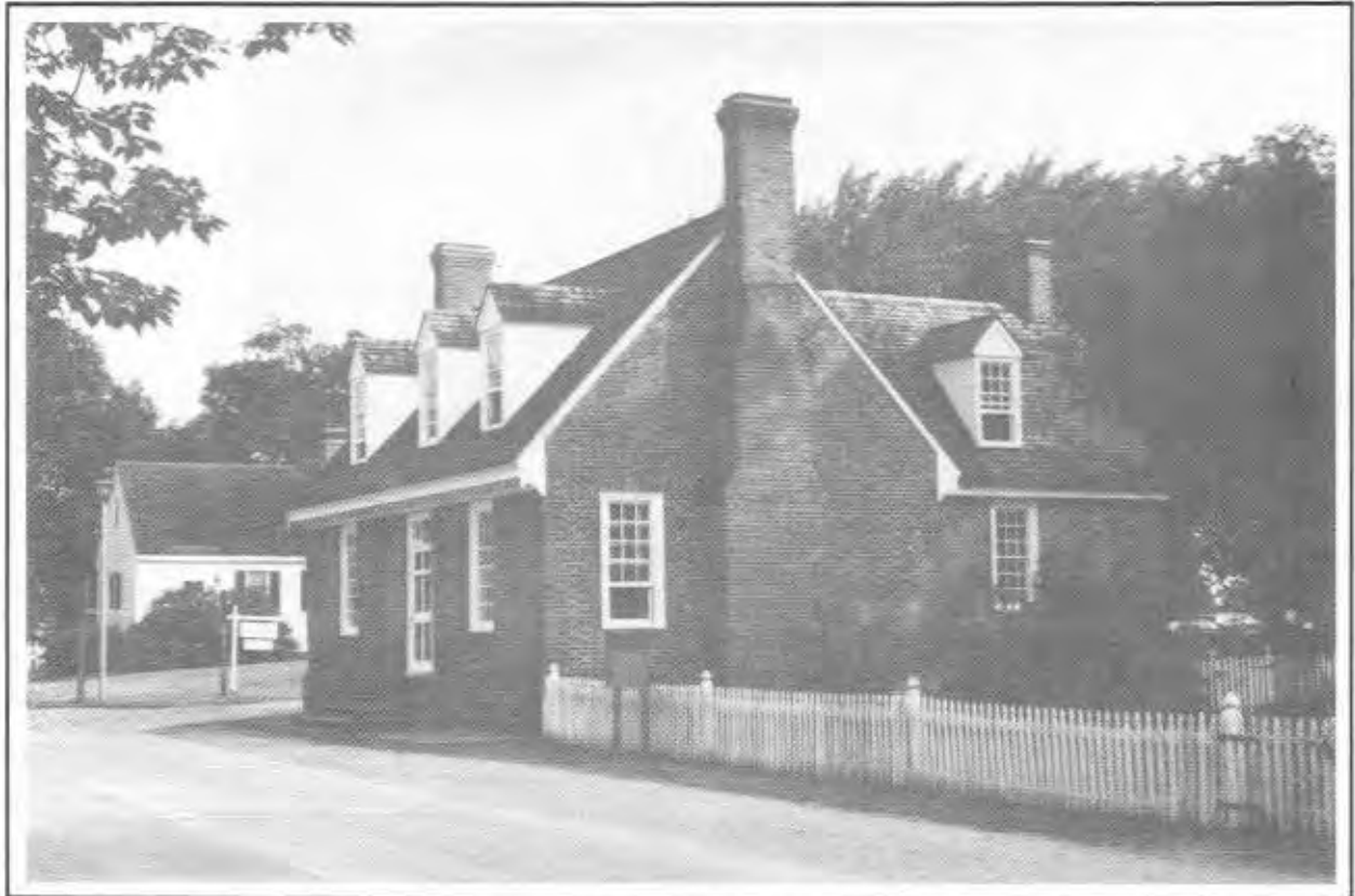
Somerwell House, Main Street, Yorktown. Home of ferryman Mungo Somerwell, this house survived the 1781 siege.
