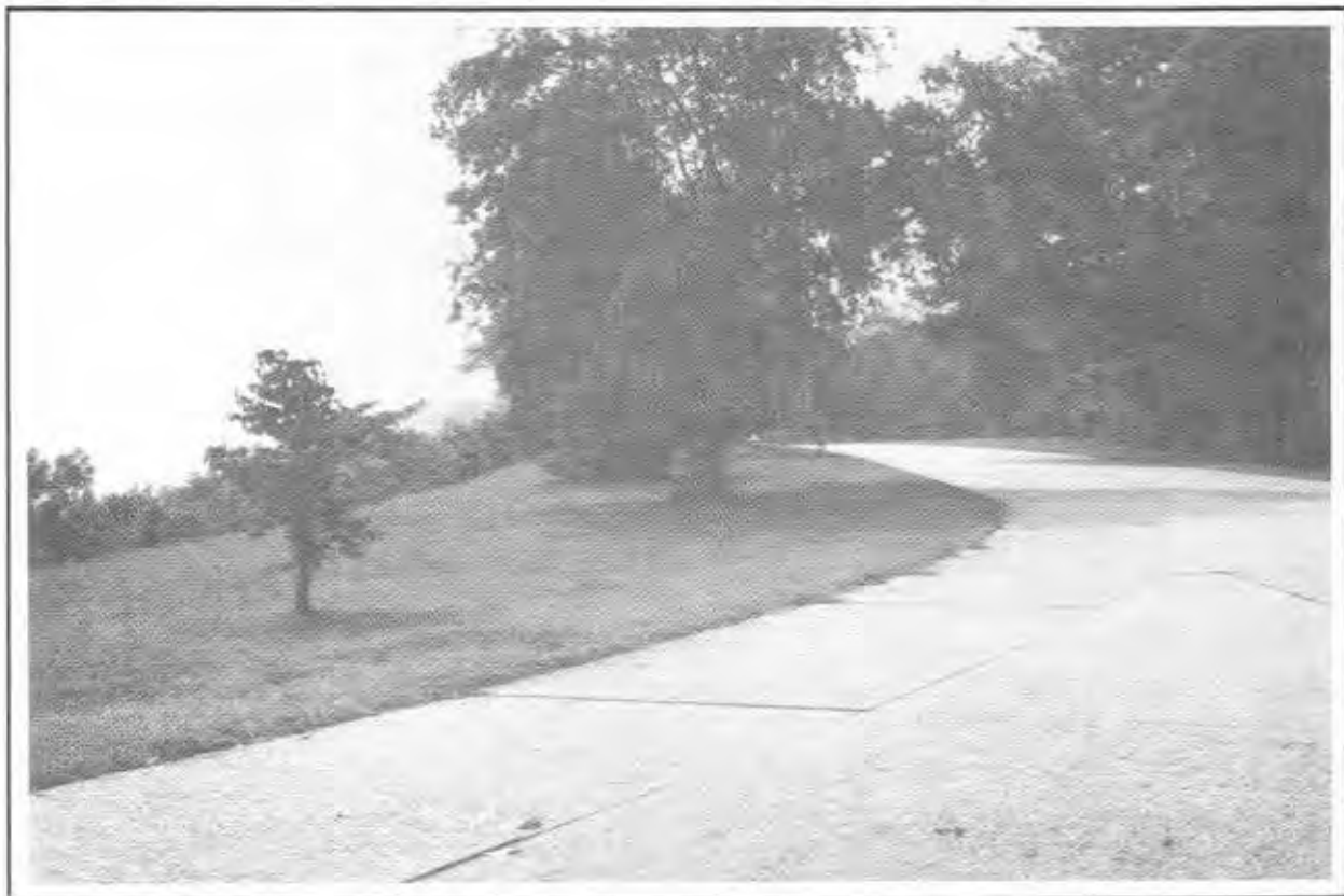
A portion of the Colonial Parkway
