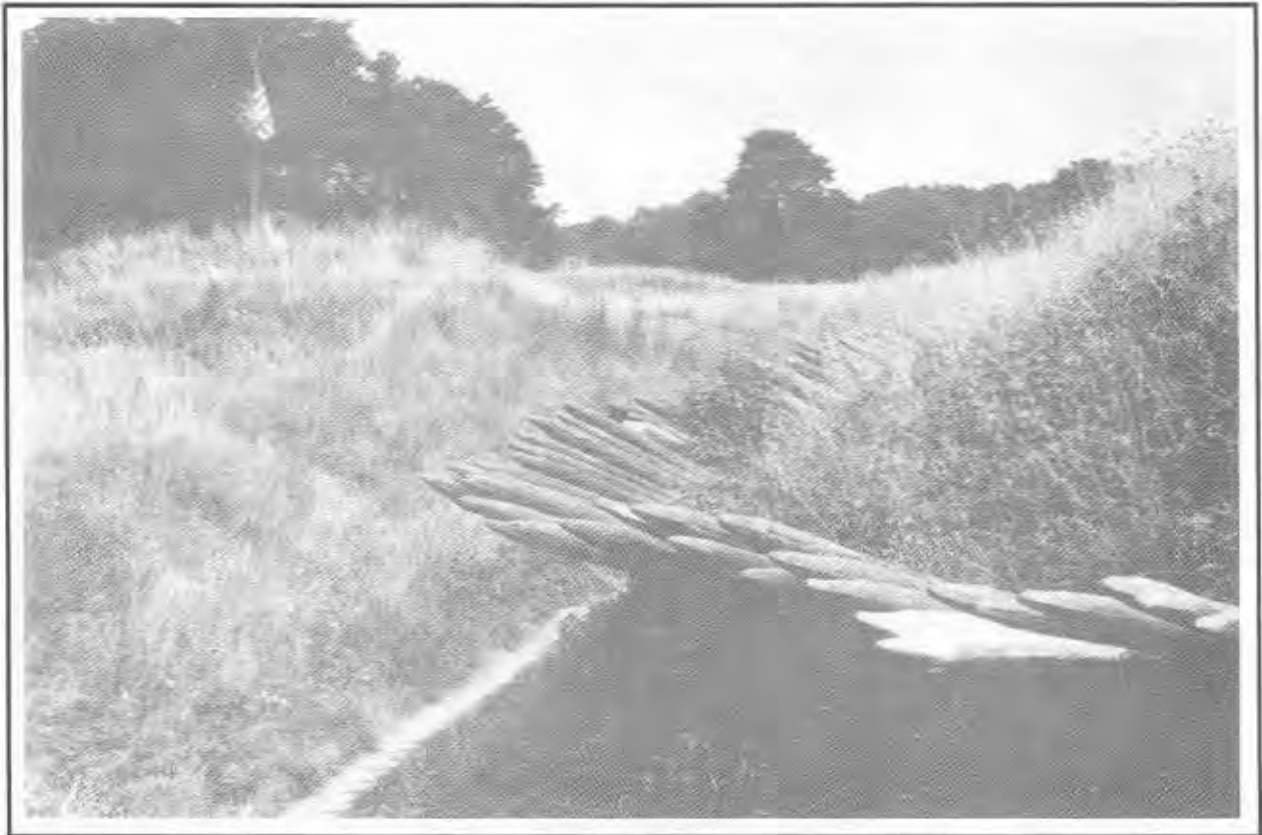
Earthworks: Redoubt with fraises, Yorktown Battlefield. Fraises, the sharpened sticks protruding from the earthen redoubts, were a more sophisticated version of abatis , or felled trees whose sharpened limbs were pointed toward the enemy, which were sometimes used in the 18th century.
