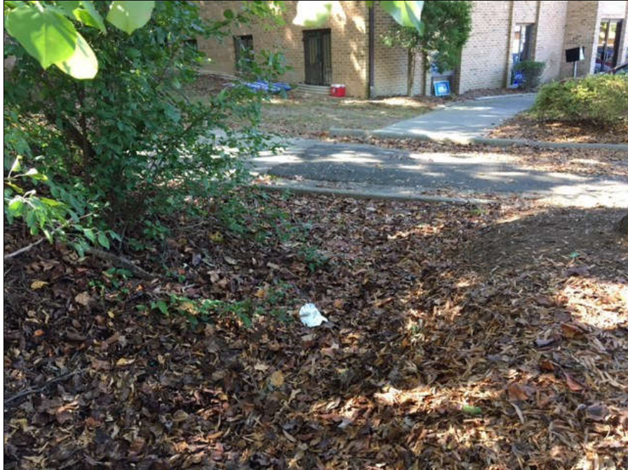
19 - Endpoint of Water A Toward Adjacent Property
