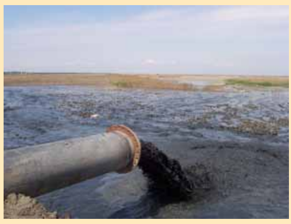
C Material flows down-slope to the west, depositing the heaviest particles first
