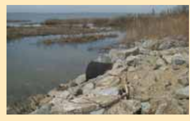
E The clarified water is returned to the James River through outflow pipes
