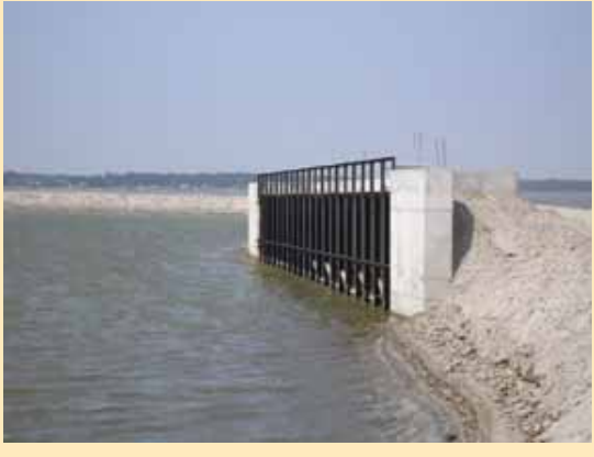
E The clarified water is returned to the James River through outflow pipes
